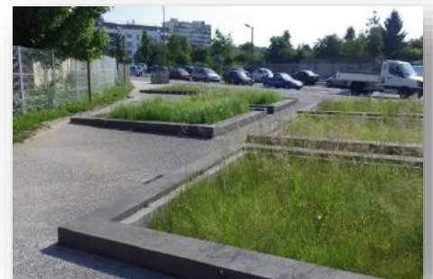
FIGURE 5 - FILTRES A SABLE PLANTES (SOURCE : DEA)
