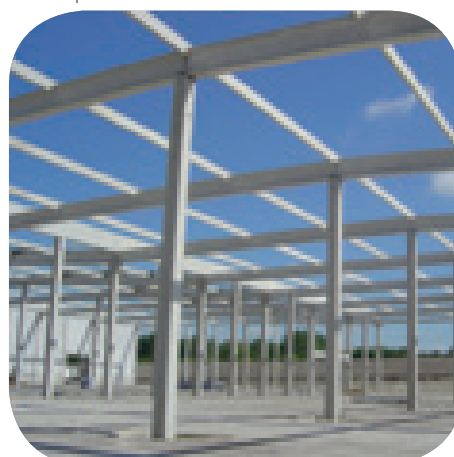
Charpente en béton, Concerto, Mer (41) Concrete framework
