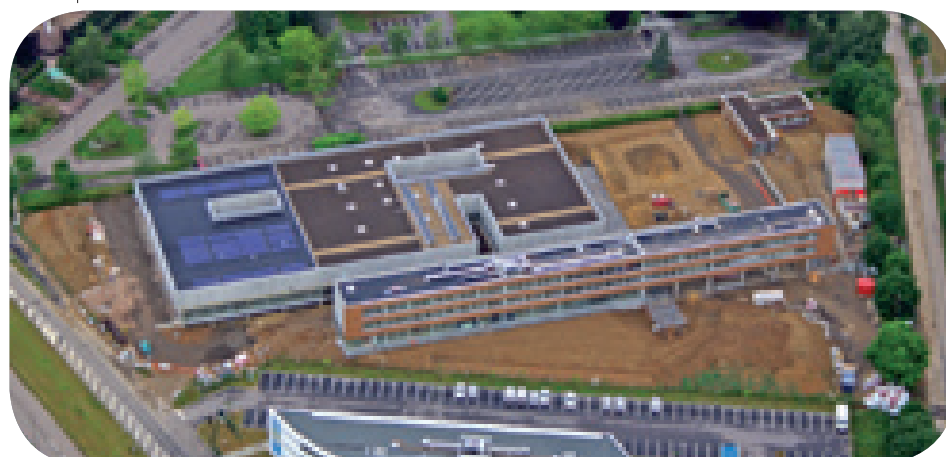
CFA Hôtelier, Metz (57) Arch. : Ropa Architecture Hotel Technical School
