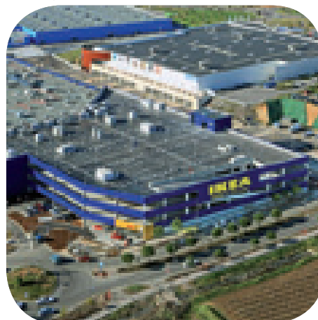
Extension et parking - IKEA, Montpellier (34) IKEA expansion and car park
