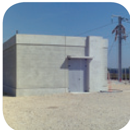
14 bâtiments techniques - Equipements de signalisation, LGV Rhin-Rhône Dijon/Mulhouse Technical buildings - Signaling equipments
