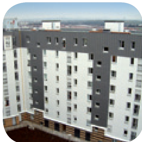
Réhabilitation de logements , Garges-lès-Gonesse (95) Arch. : Arcane Housing renovation
