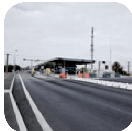
Aménagements VRD - Gare de péage, Thelus (62) Tollgates land improvement and roads
