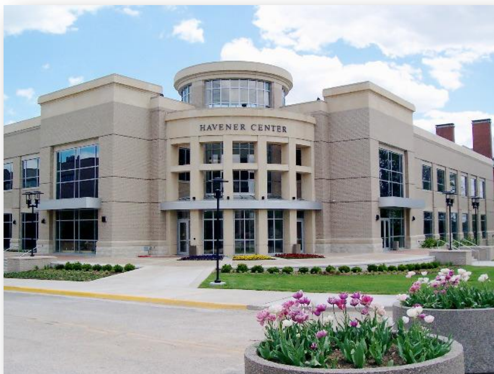
External picture of the Havener center of the University of MS&T
