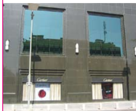
Centre commercial - Salhiya
