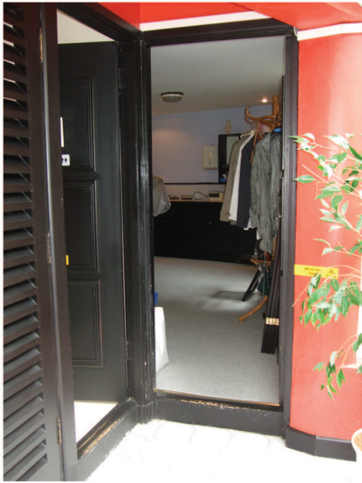
Bathroom and Consulting room Entrances
